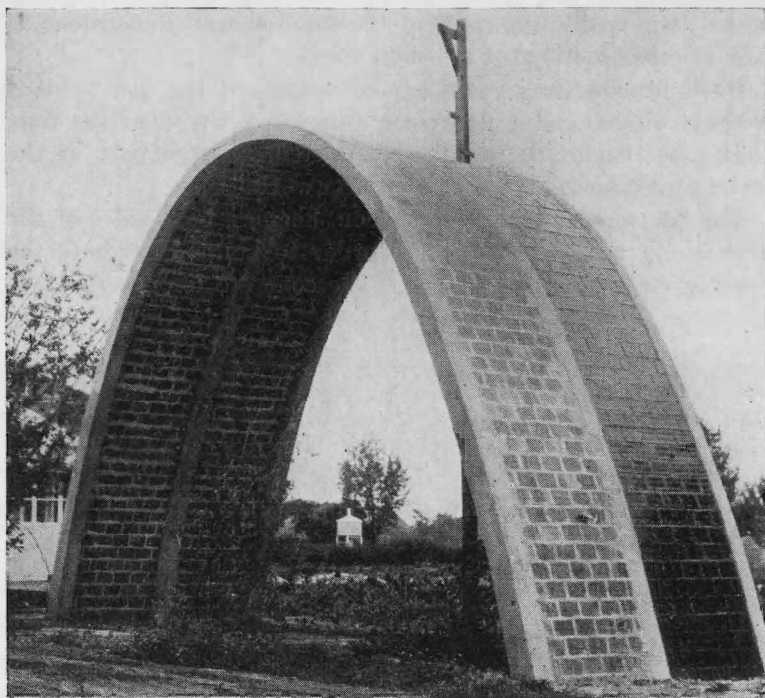
Fig. 26. The completed section of the full sized arch.
